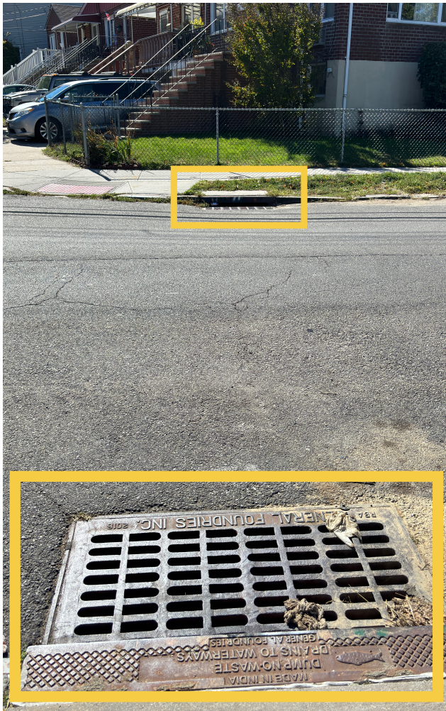
Figure 17. 2 of 5 catch basins on Poppenhusen Ave, at intersection with College Place.
