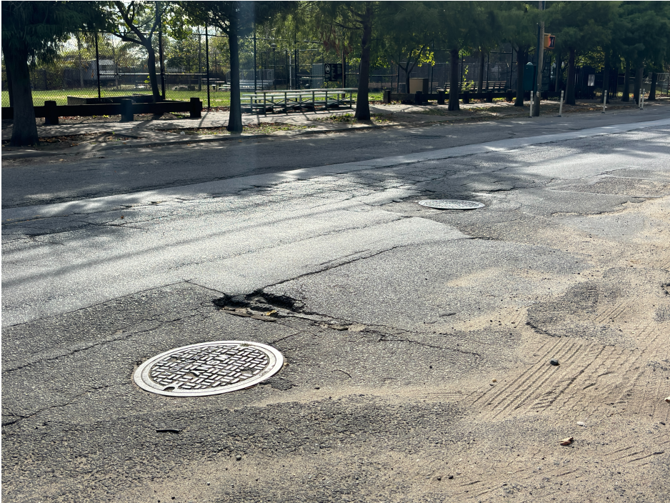
Figure 21. 2 manholes on 147th Ave by Brookville Park.
