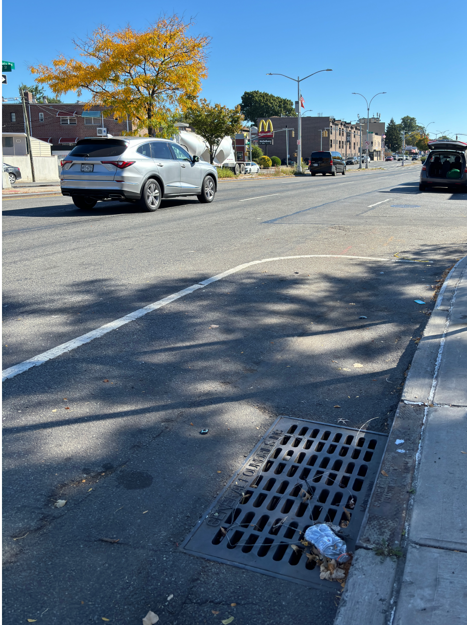
Figure 15. Catch basin on Astoria Blvd, adjacent to 87th St.
