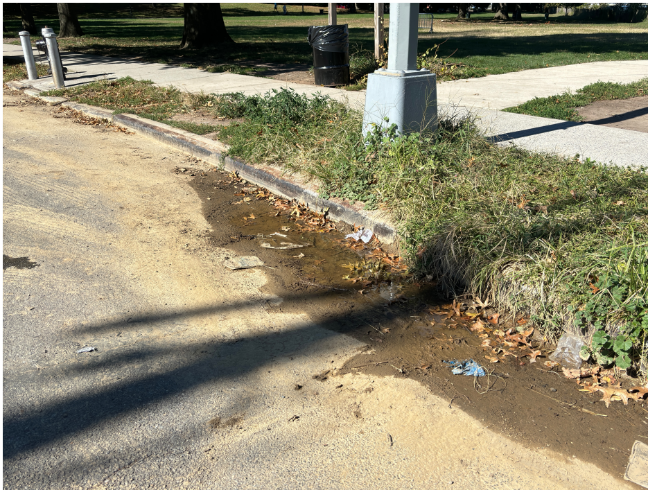
Figure 22. Ponding in College Point on Poppenhusen Ave, by Hermon A. MacNeil Park. A curb strip is raised just above the area with ponding.
