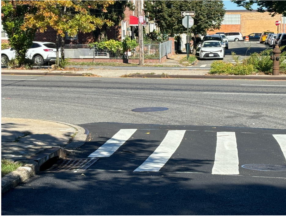
Figure 16. Catch basin on 86th St off Astoria Blvd.
